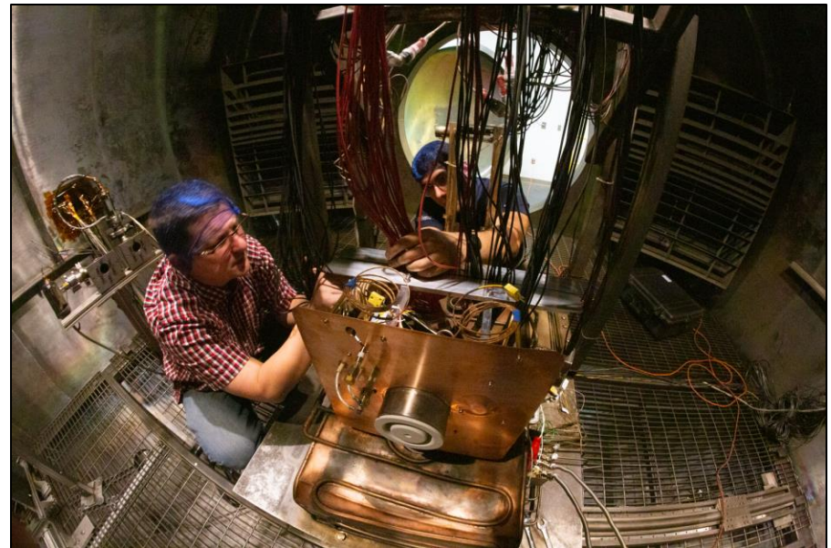
HET-X experimental installation
